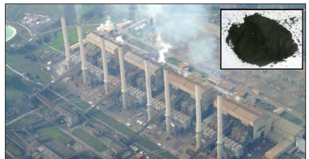
At the power station, coal is crushed into a powder so it can burn faster
