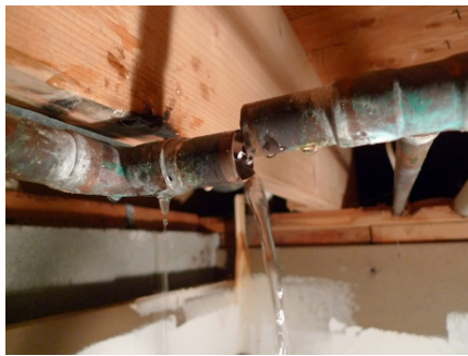
LEAKING PIPES AND TAPS
